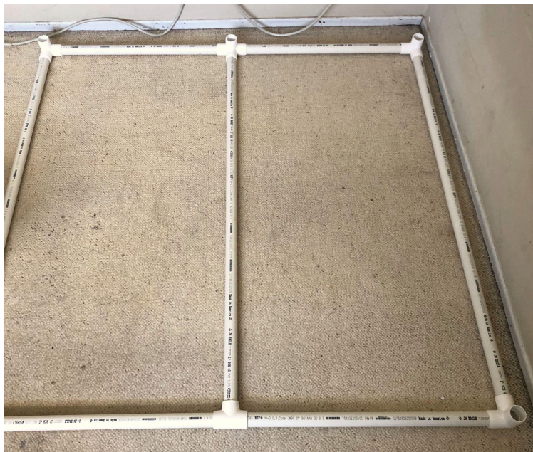
Step 2 - Ceiling strut built into the ceiling panel. The front of the booth is closest to the camera. Notice there is a "T" connector on the front and a "K" connector on the back
