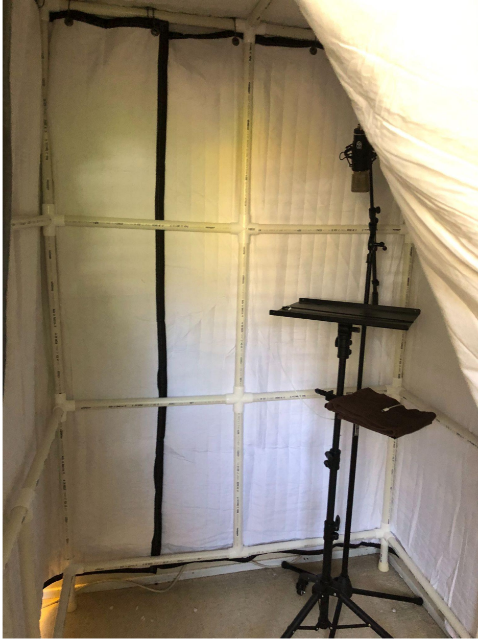
Booth blankets in place. View from front door flap area. Roughing in position for microphone stand, laptop stand and accessories.
